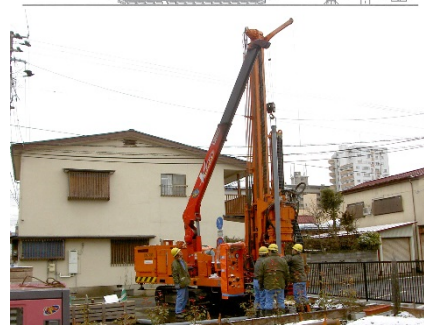
Water well drilling
