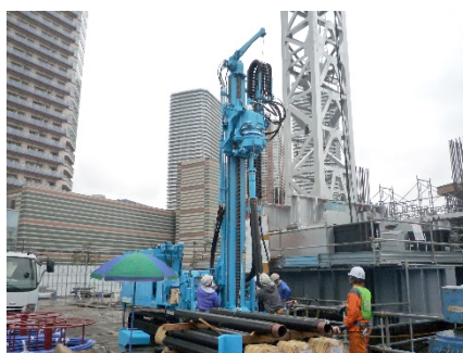
Geothermal hole drilling
