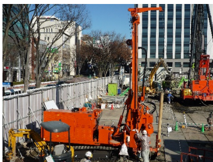
Geothermal hole drilling
