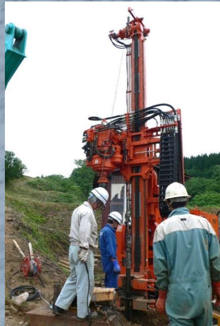
Investigation drilling for land slide restraint
