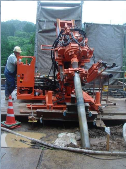
Anchoring for land slide prevention
