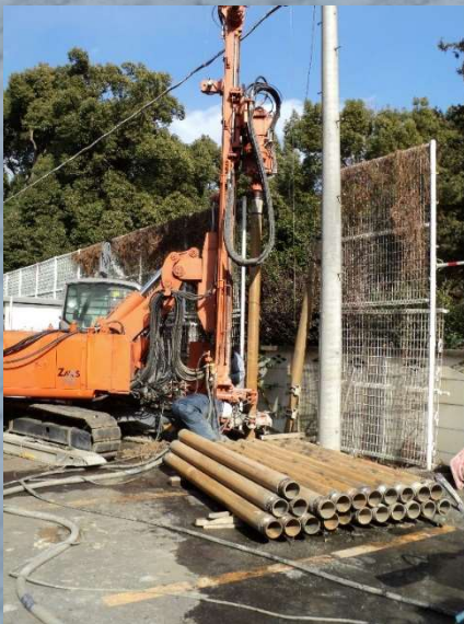
Drilling of underground geothermal hole at international school
